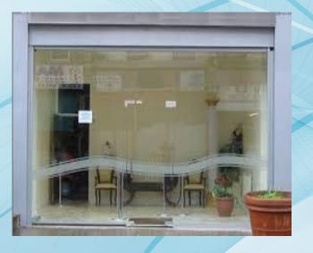
Glass partition with 10/12mm toughened glass and laminated toughened glass with options of swing and sliding doors. Full height partition and half height partitions for commercial & residential layouts. Transparent and opaque overviews can be obtained with sand blasting and stickering
