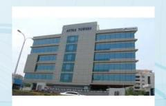
Aluminium Composite cladding or ACP is typically a metal curtain wall system.ACP is made from lightweight Aluminium with Hard Insulation.With a huge selection of finish types and colours.ACP is used for exterior claddig, column covers, interior wall and partition panels.
