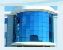
Facades or Curtain wall system combines glass ,either transparent or spandrel or both ,and vertical and horizontal mullions acting as structural members to transfer wind and gravity forces to building structure. Custom or standard unitized or stick framed, double skin or fin facades, framed or frameless structurally glazed system are designed
